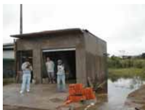
MON03PON09FOT02 - Vala natural entre lotes
